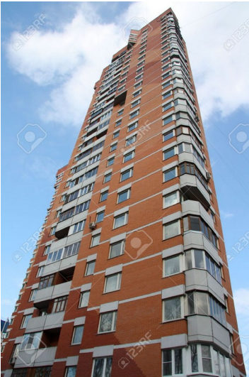
block of flats (many floors)
